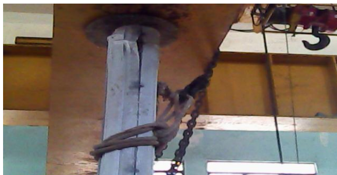
4(c). Failure of column L/D 25 at top with 3/#8
